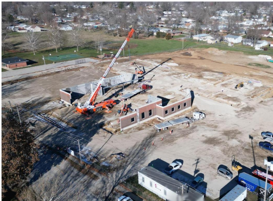
PRECAST ERECTION
